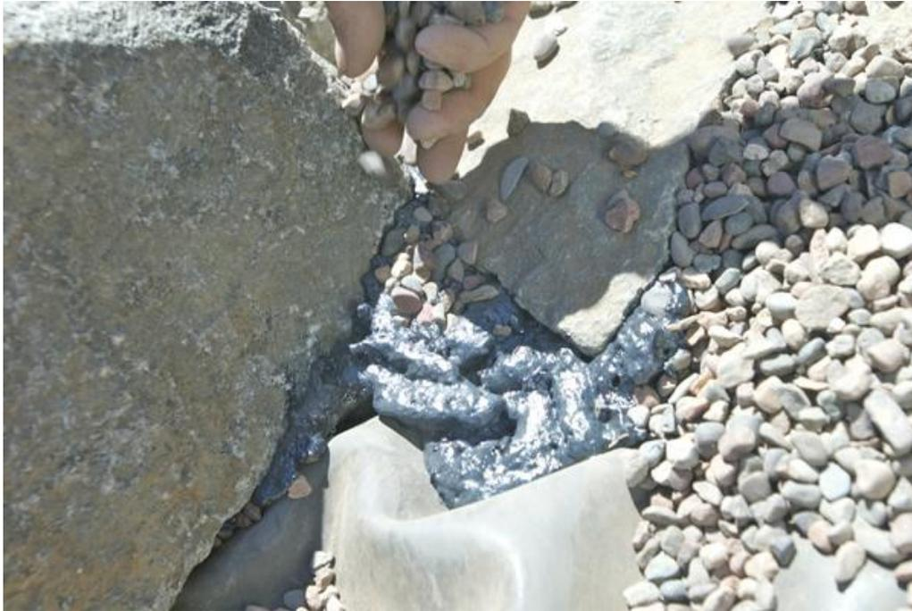
Use the can of rock foam that is included with your kit to fill in cracks between stacks of rocks. Use foam where flat rocks meet the liner to keep the water flowing above them.
