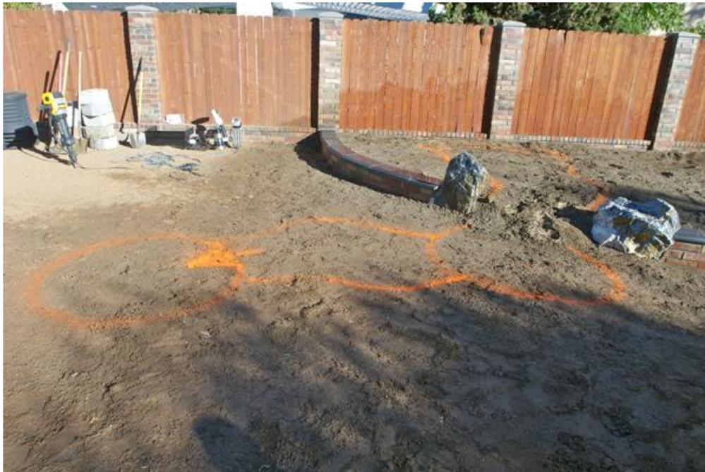
Once you have determined where you would like to place the feature you will want to mark out the position of the waterfall, the basin, and the stream if your model includes one. The best way to do this is with a can of marking spray paint from your local hardware store.
